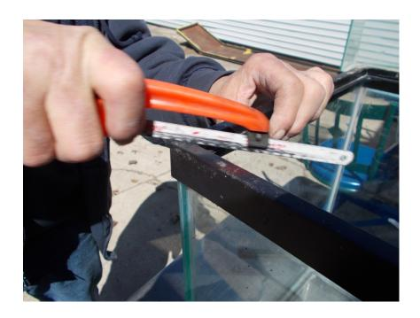
• Cut notches into the frame, inside, on top and outside of the tank as shown here
